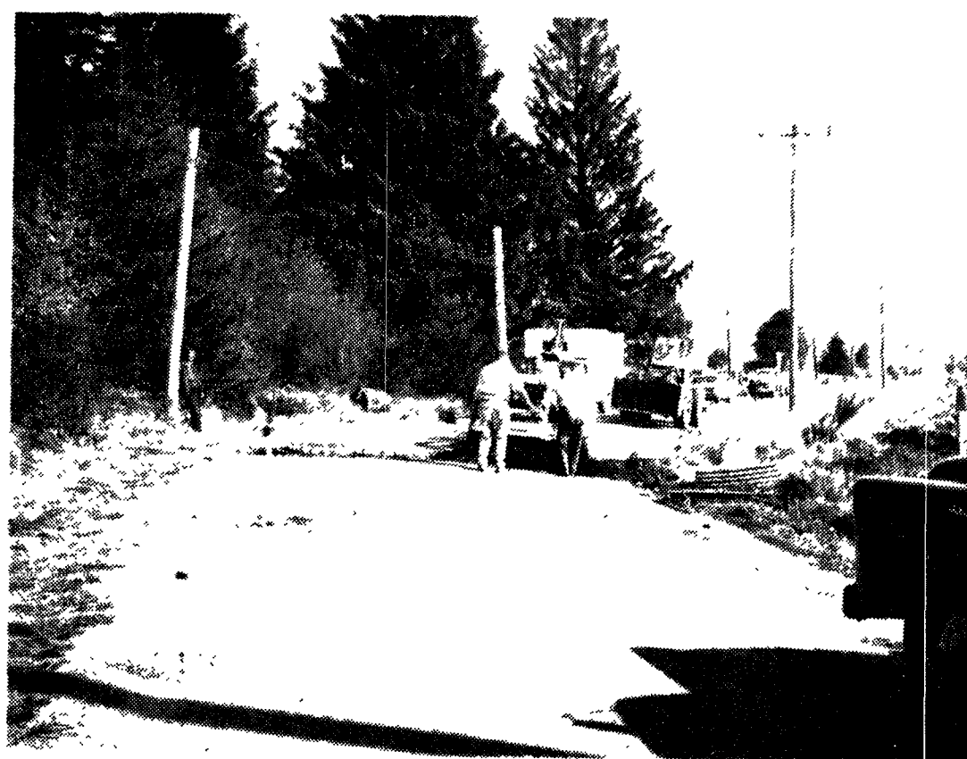
The county installed a new 4' culvert across Calawah Way last week that should solve some of the drainage problems of the past. The upper prairie area should not have the old water problem and the Kelso's chickens should be able to get thru the winter without swimming for their lives.
